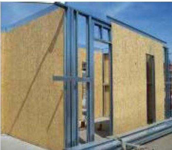
Eurocode 8 **does not provide specifications** applicable to Sheathing-braced structures
